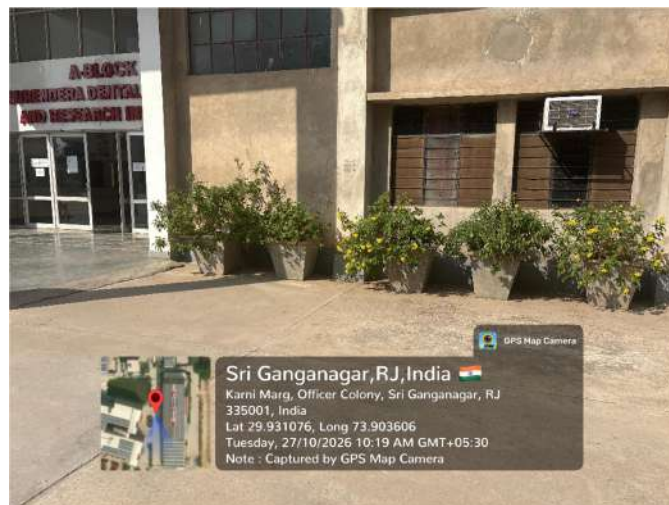
Plate 1.3: Post-Sanitation Inspection — Cleared Courtyard & Aesthetic Entrance Apron
